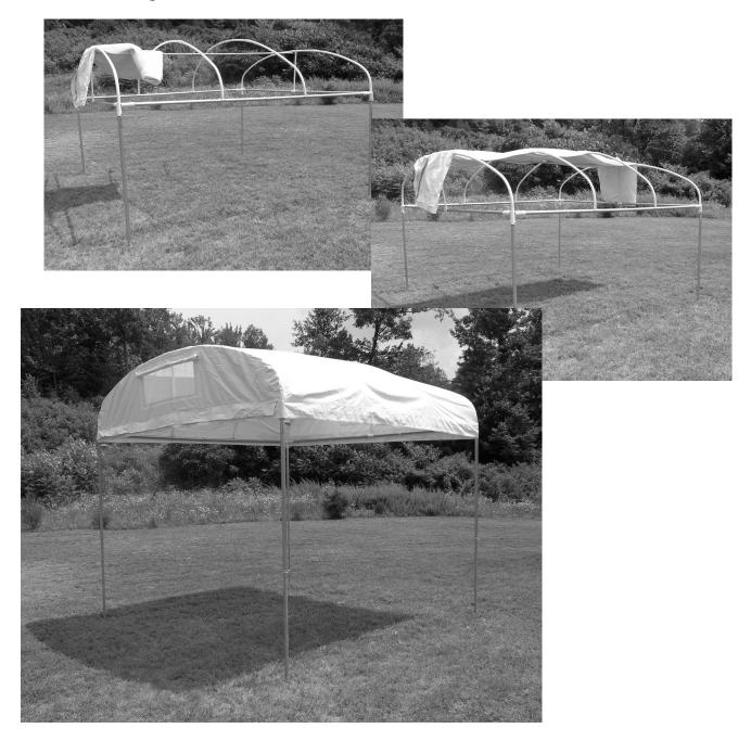
**5.** Step underneath roof and attach Velcro straps to Side and End Rails, then reach up and attach Velcro straps to Rafter arches.
