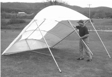
Canopy roof raised and supported on telescoping leg pole
