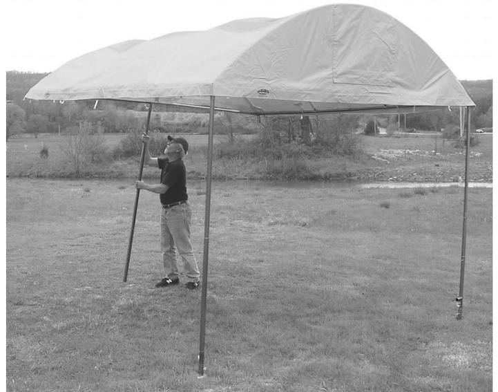
Pushing frame up using the Rear Door Leg
