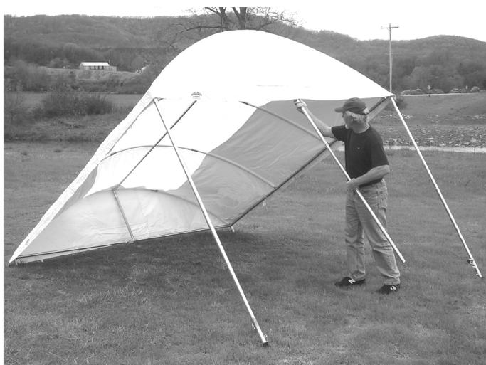
Front legs attached, removing the EasyRiser Pole
