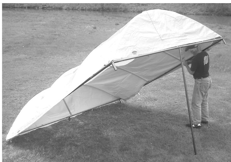
Canopy roof raised and supported on front EasyRiser pole
